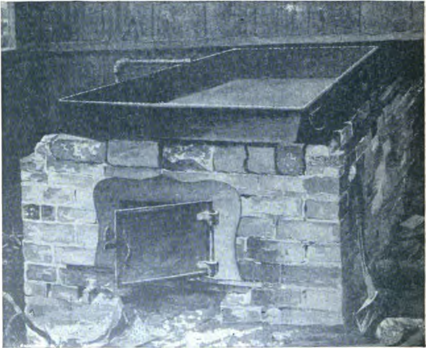
Fig. 28. An old time evaporizer for making maple sugar still in use in Ohio.
